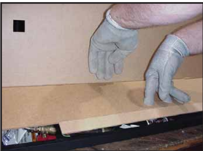
Figure 13.12 Opening Lower Access Panel
